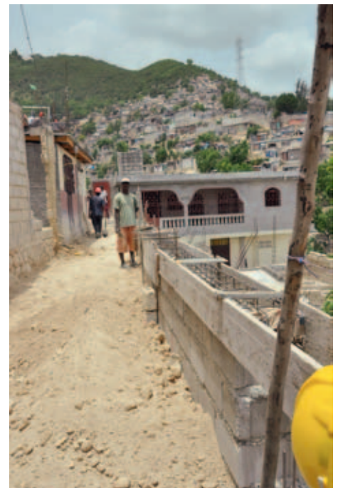
Paved Road as Part of Rehabilitation Project in Haiti (Photo by UNDP)
