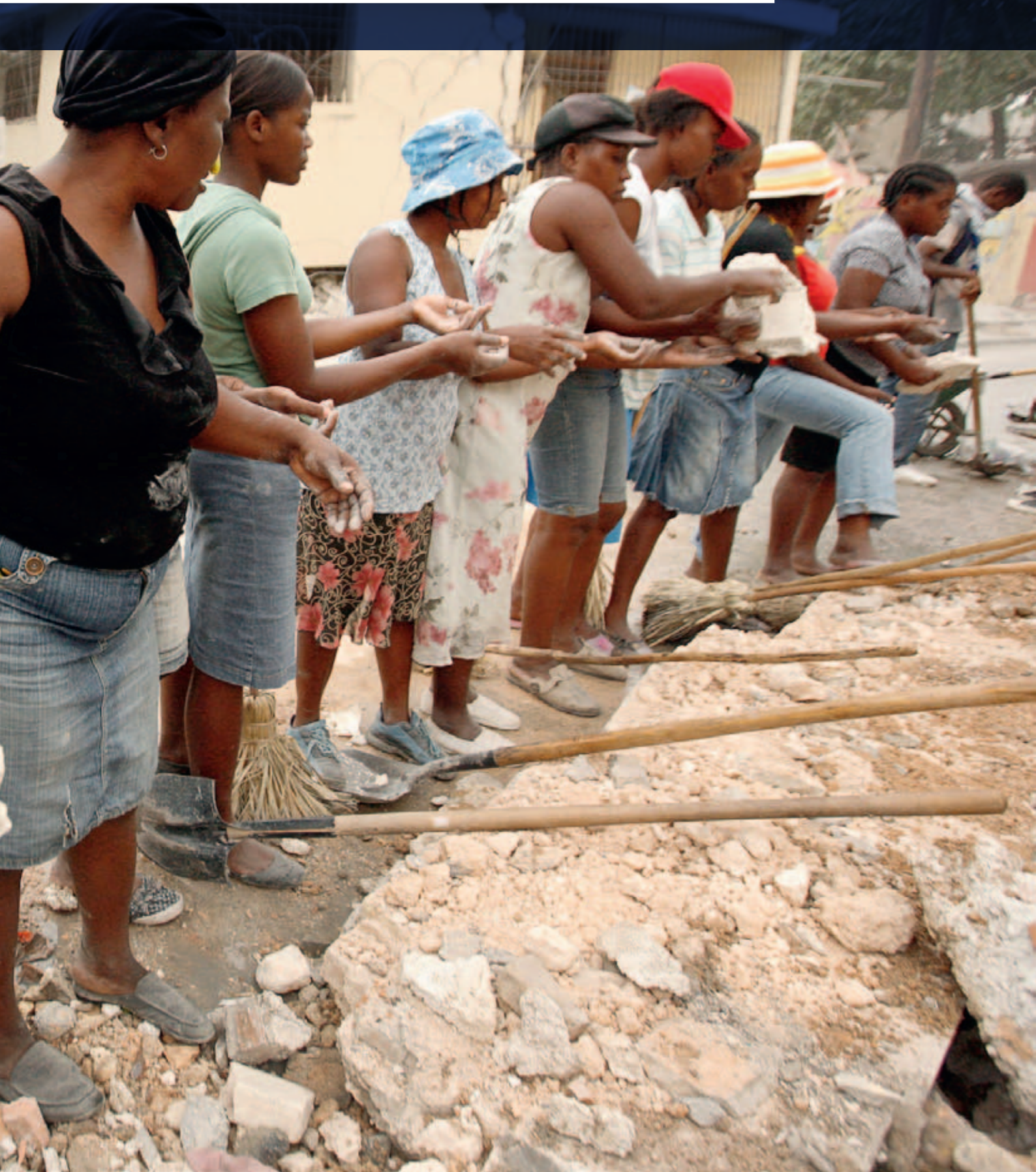
Men and Women Cleaning the Rubble as Part of Cash for Work Programme in Haiti (Photo by UNDP)
