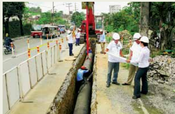
New pipes are laid to increase water and sewage system capacity.
