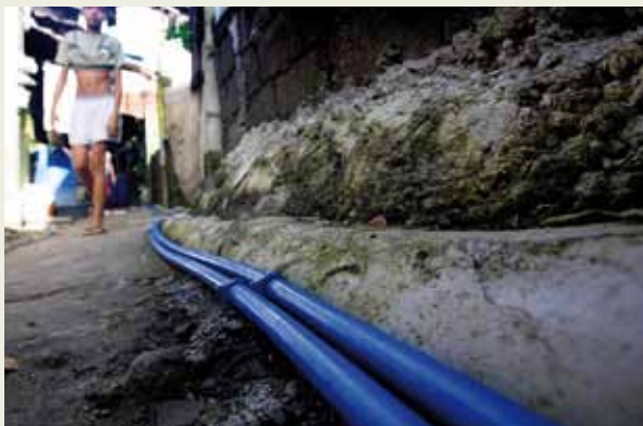
Manila Water is upgrading infrastructure in slum areas in compliance with its concession contract.
